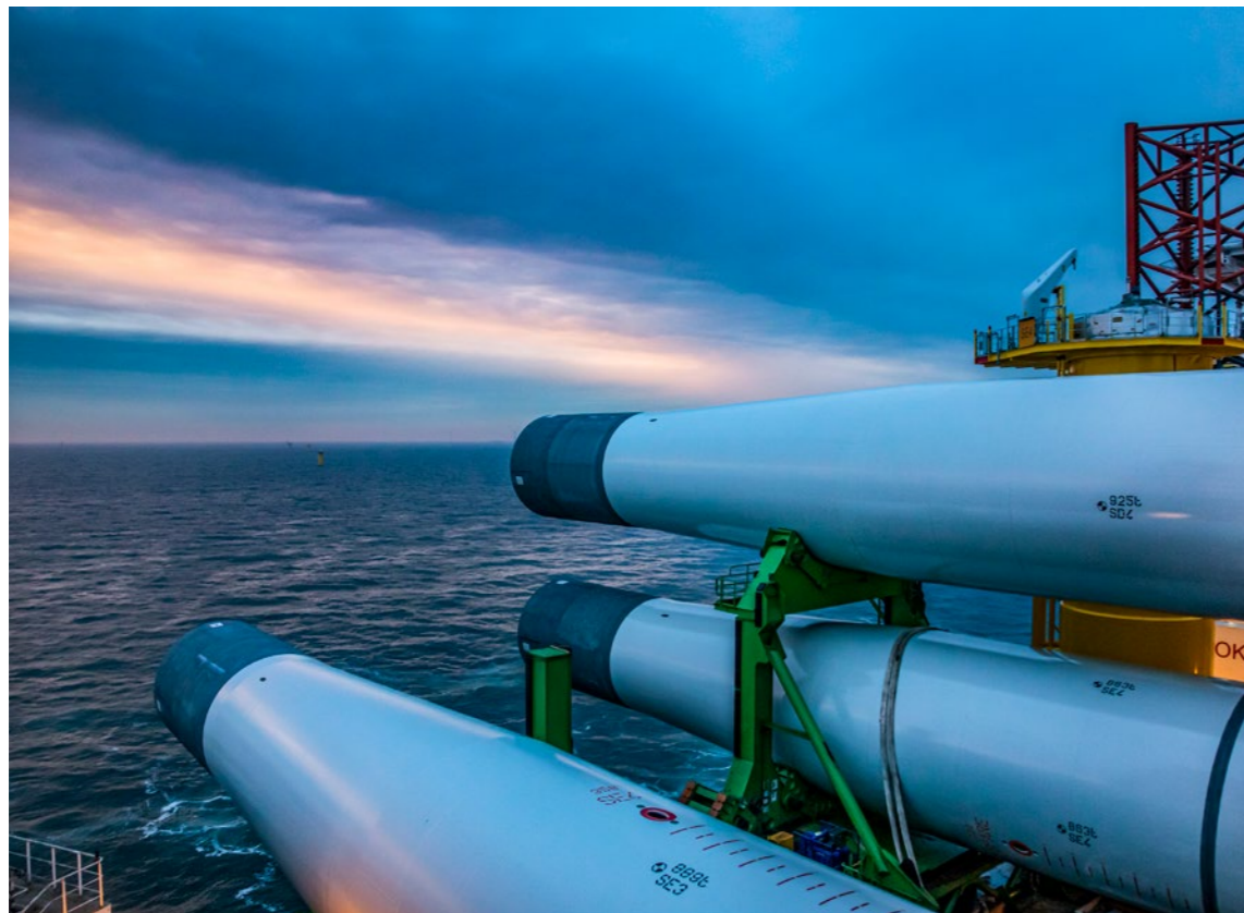
FRANCE We will undertake the transport and installation of the monopiles and transition pieces for the first offshore wind farm ever to be installed in France
